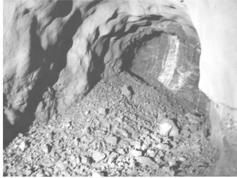
**Fig.5** Shape of fragmented rock after blasting.
