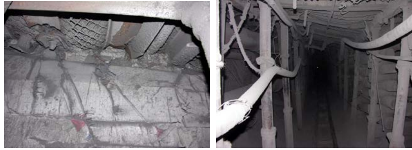
(a) Filling wall
